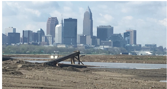
Water is added to dredged sediment via barge and hydraulic pumps, like the one shown here. This slurry then makes its way through a series of settlement ponds and water control structures so that the sediment falls out of suspension and settles within the facility.
