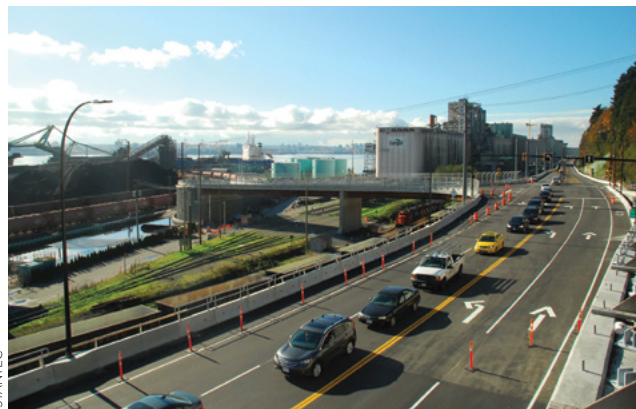
The Low Level Road Neptune Cargill Overpass.
