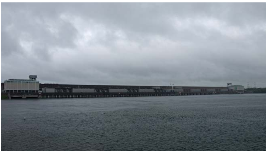
The Moses-Saunders Power Dam near Cornwall, Ontario.
