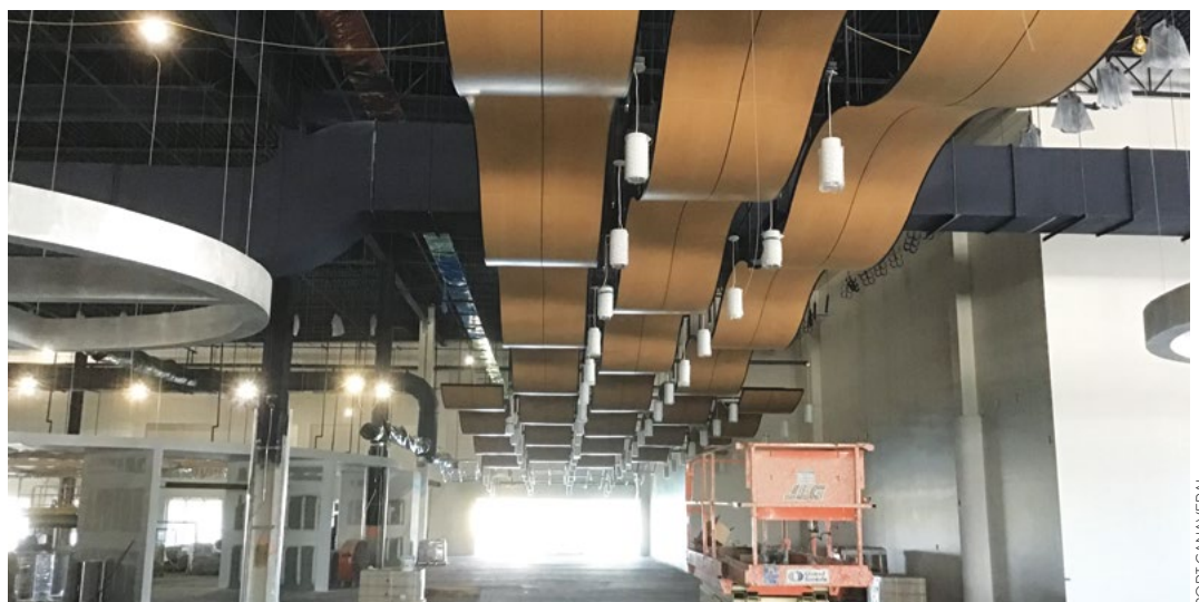
CT3 Interior ceilings.
